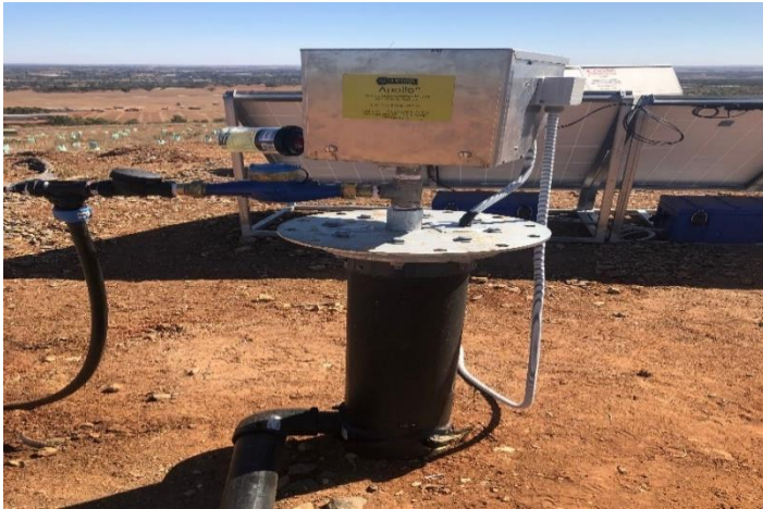
Figure 2: Blackhawk Solar/Battery powered leachate pump installed at Uleybury Landfill Renewable Energy Park
