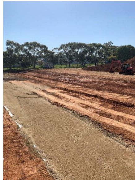
Relocated swale drain
